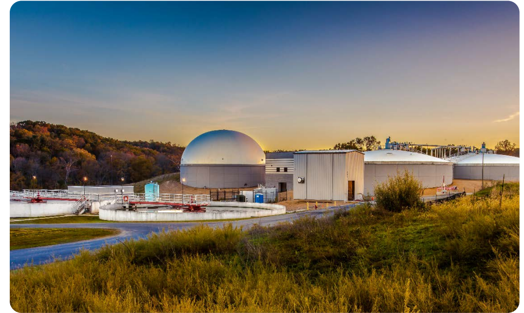
ESG Project: Frederick-Winchester Service Authority, Virginia
